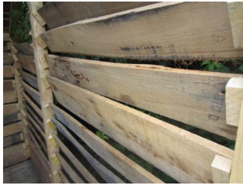
Bespoke sun screens for balconies.
